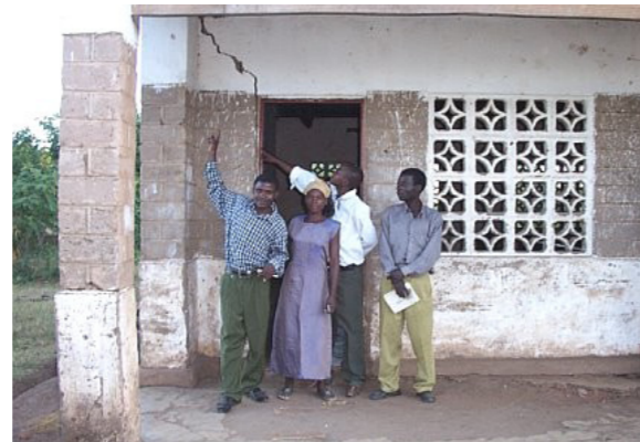
Teachers from Chikunkha point out damage to the school wall.
